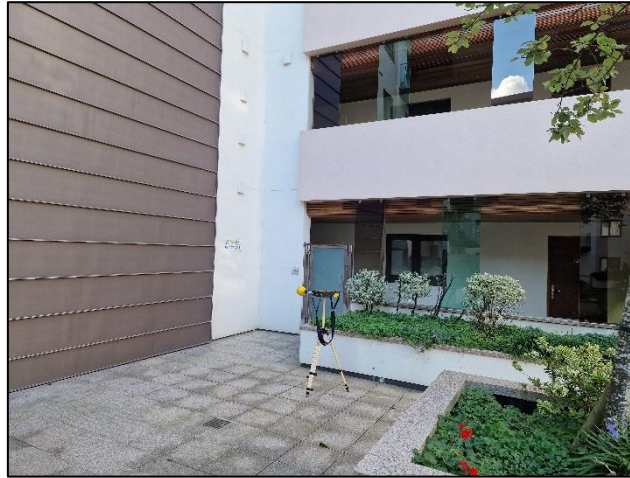
Figure 2 – Location of the peak where emission levels were measured.
